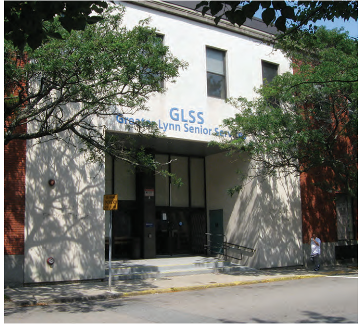
Front entry of 8 Silsbee Street in downtown Lynn where Phoenix Food Hub programs and food pantry will be located. A redesign of the first floor space is underway.
